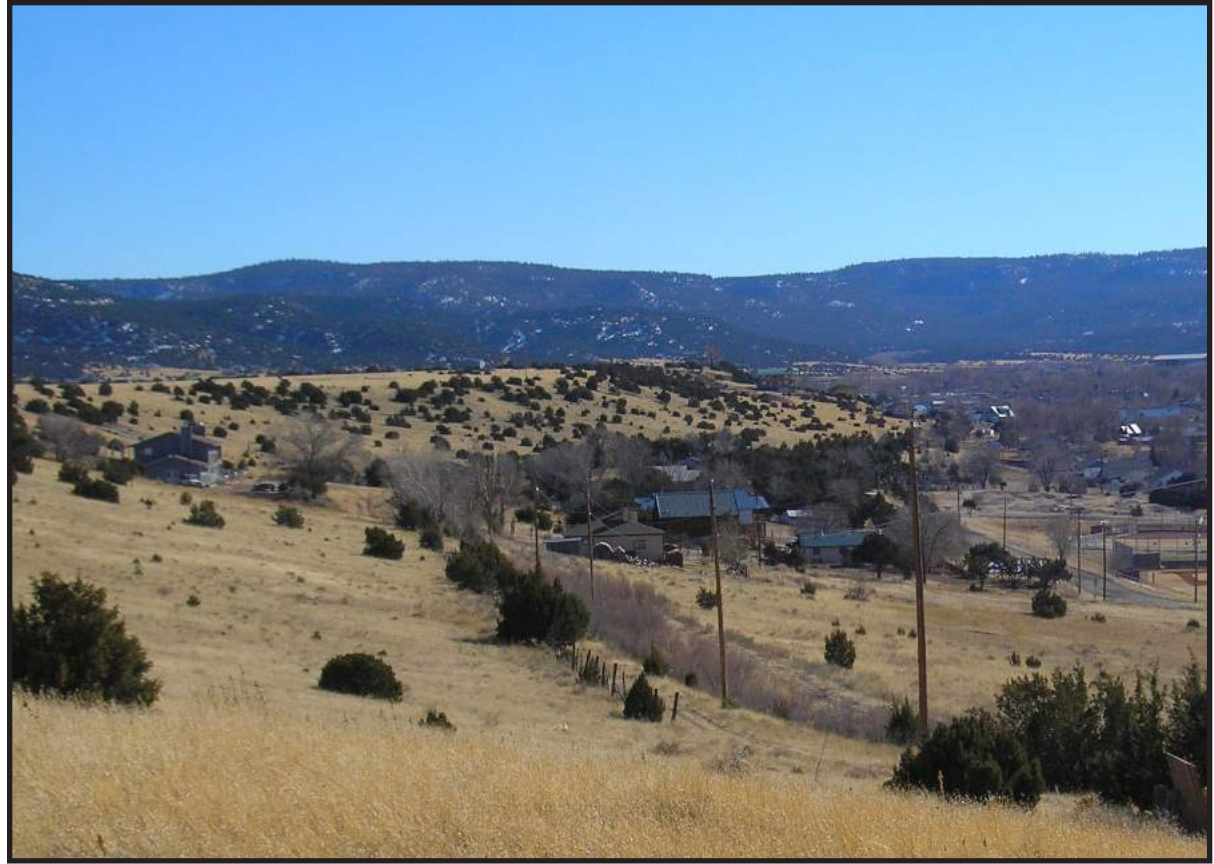
View to the southwest from the top of Central Park, along the north end of the proposed Ridgecrest Trail. Across the center of the photo is the current Amity Ditch which will become a hiking and biking trail.
