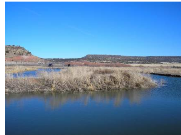
Wastewater treatment ponds, Springerville, Arizona
